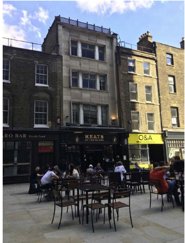
FIGURE 15.4 Café culture in former road space in the City of London, UK.
